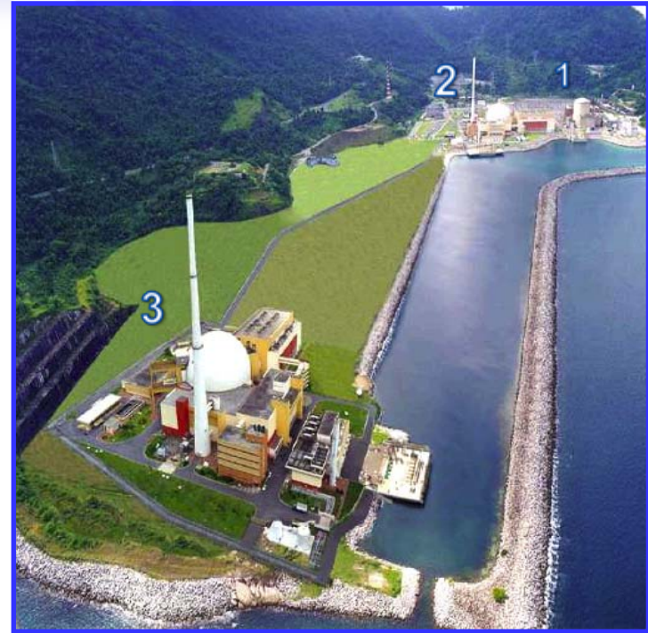
Angra 1 – start construction 1971 - operation ( 626 MW e ) Angra 2 – start construction 1977 – operation 2000 (1229 MW e ) Angra 3 - most components purchased in 1995 but has been in storage ever since, consuming 50 million dollars a year in maintenance costs.
