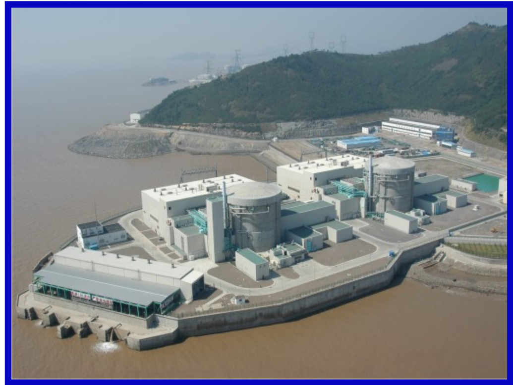
Qinshan Nuclear Power Phase III Project (China)
